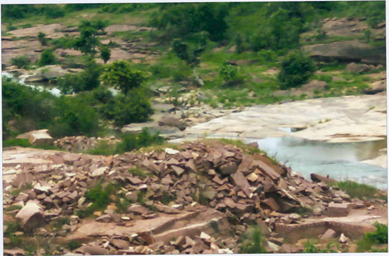
Excavation & dumping of Over burden near River side
